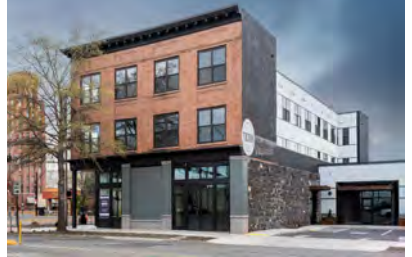
Façade - Southwest View
